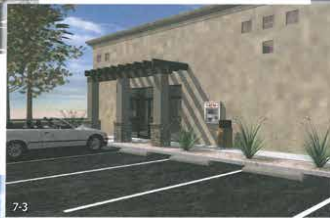
Building 5 Lattice and Features Detail
