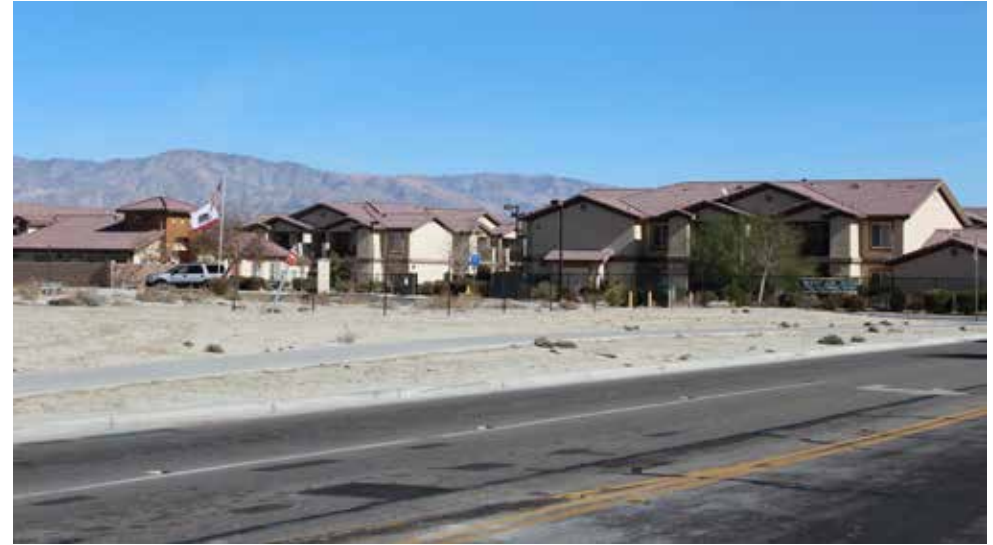
Heritage Park Senior Apartment behind subject site (some interior roads shared)
