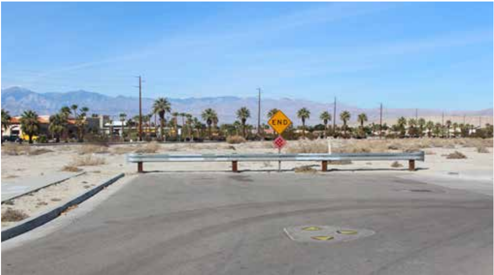
End of sidewalk and curb back of the subject property near apartment project
