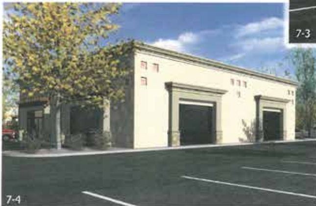
South West corner of Building 5
